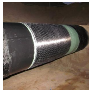
5.step: finished installation of pcw -ready for final isolation
