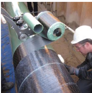
spirally wrapped application- MAOP reinforcement of whole pipe segments
