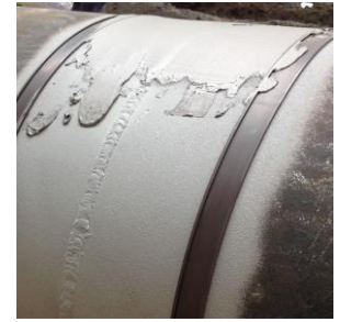
2.step: equalisation of dents, ext. metal loss or girth welds with pcw -filler material
