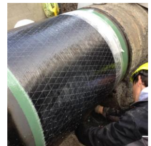
4.step: application of the pcw (permanent carbon wrap) with pcw -winder
