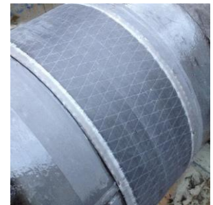
5.step: finished installation of pcw -ready for final isolation
