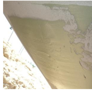
2.step: equalisation of dents, ext. metal loss or girth welds with pcw -filler material
