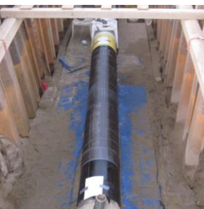
spirally wrapped application- MAOP reinforcement of whole pipe segments
