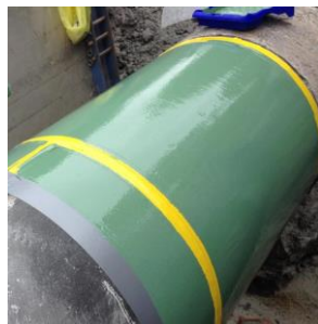
3.step: base coating with pcw -primer or pcw -filler for galvanic separation
