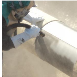
1.step: greaseless surface preparation (grinding or sandblasting acc. to specification)
