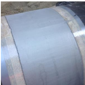
3.step: base coating with pcw -primer or pcw -filler for galvanic separation
