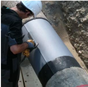
1.step: greaseless surface preparation (grinding or sandblasting acc. to specification)
